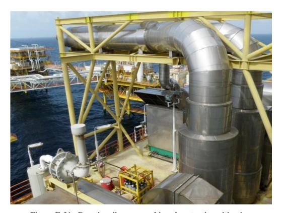
Figure E-21: Reactive silencers used in exhaust noise mitigation
