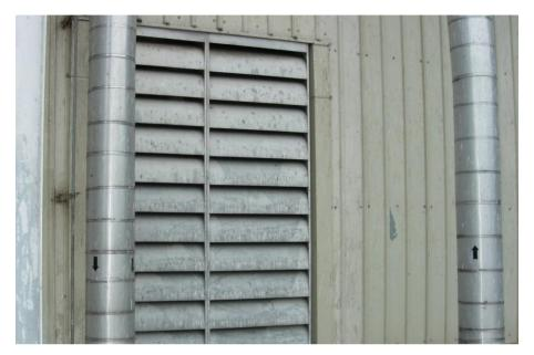
Figure E-22: Acoustic louvres used for natural ventilation opening in power station turbine hall
