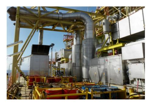
Figure E-14: Full enclosure for power generating sets
