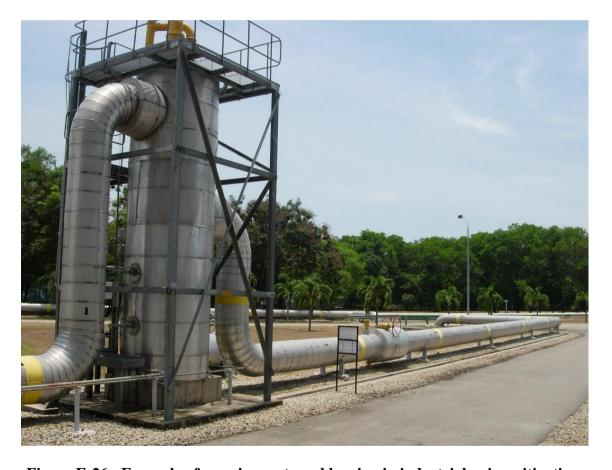
Figure E-26: Example of gas pipes external lagging in industrial noise mitigation
