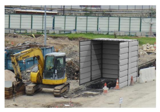
Figure E-18: Movable partial enclosures for construction works noise mitigation
