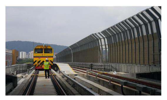
Figure E-7: Metal noise barriers used in railway noise mitigation
